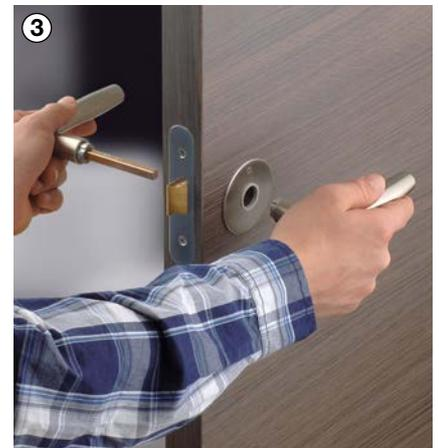
3 Put the door handles together and fitting is complete! (if necessary, stick on the escutcheons)
